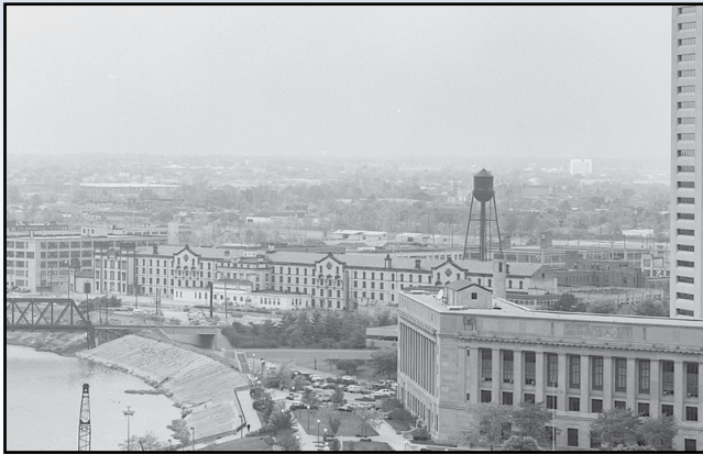
1989 elevated view of south face of Ohio Penitentiary
